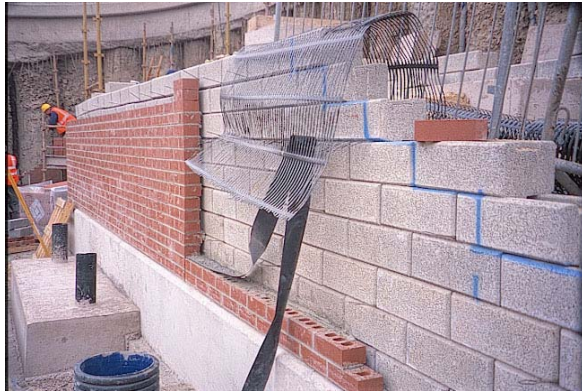
Fig 1: TW, Link Wall at Pallion
