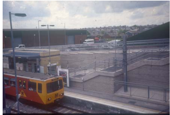
Fig 2: TW, Standard Wall at Millfield Station
