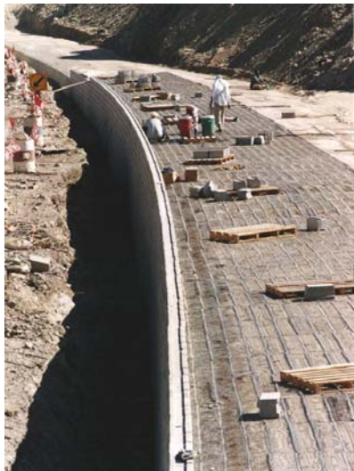
Tensar Wall system built in harsh desert conditions with heights over 18m.
