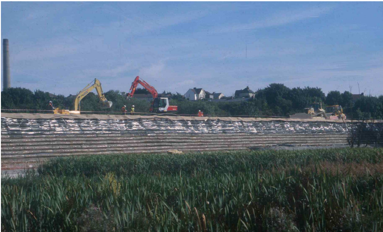
Constructing the GreenSlope face of the steep 8m high railway embankment
