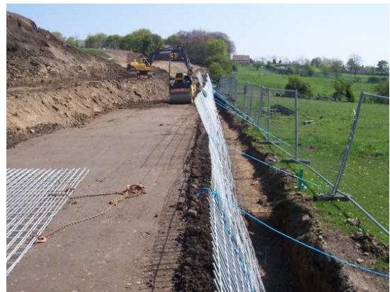
The TR2 system needs very little temporary support.
